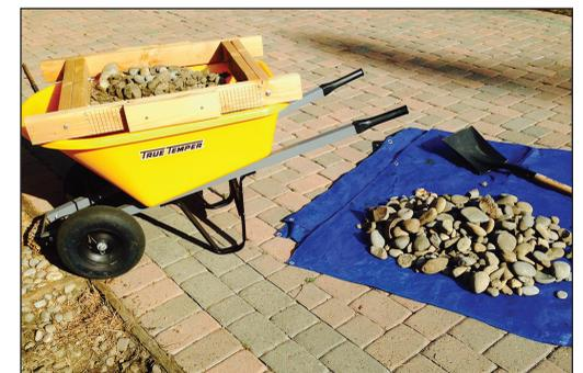
Driveway gravel infiltration systems require annual maintenance to remove fine sediment from debris and road abrasives. The best way is to remove clogged gravel, sift it clean in a mesh tray over a wheelbarrow and return the clean rock back to the gravel infiltration system.
