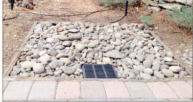
To facilitate maintenance, sediment traps for driveway gravel infiltration systems collect sediment in the trap before it flows into and clogs the gravel.
