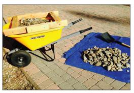
Driveway gravel infiltration systems require annual maintenance to remove fine sediment from debris and road abrasives. The best way is to remove clogged gravel, sift it clean in a mesh tray over a wheelbarrow and return the clean rock back to the gravel infiltration system.
